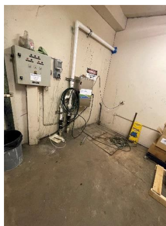
Existing sewer pump station.
